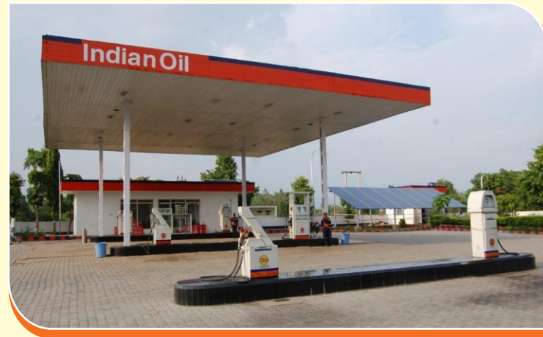
IOC's Solarized RO: M/s RKBK, Dariba, Raibareilly, Uttar Pradesh
