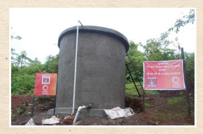
connected to each household from the water tank set up at an elevated location from where water is released through gravity. Water pumps are installed near the recharge pit to pump water up to the water tank.
