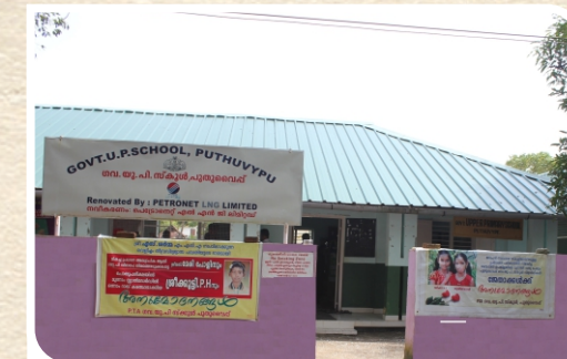
"Renovation of School Building"
