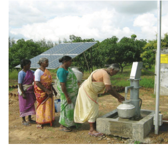
Solar Water Pump.
