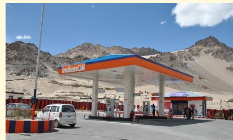
Solarised Lotus Zangpo Memorial Filling Station, Leh
