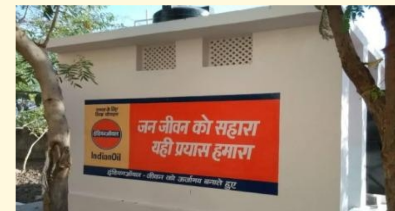
Toilet constructed by IOC at Govt. Primary School, Vasodara, Ahmedabad, Gujarat
