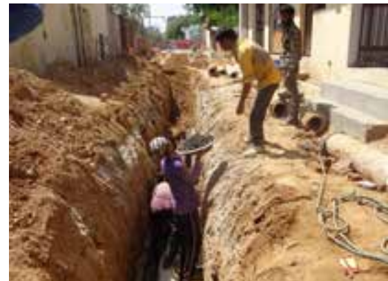
Sewer lines being laid in Manesar
