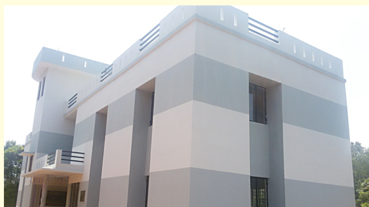
New Boys' Hostel constructed by Cochin Shipyard Limited at the School
