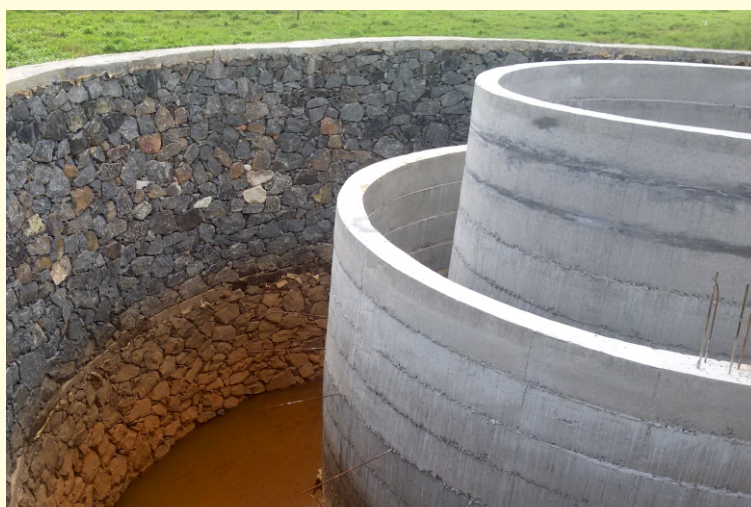
Three Layered Water Filter cum Collection Tank constructed under CSR of CSL
