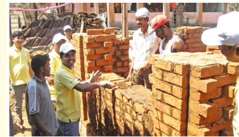
Employee volunteers constructing house for the poor at Karjat, near Mumbai
