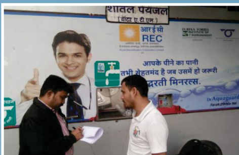
Installation of Water ATM at bus stations of Uttar Pradesh to provide safe drinking water
