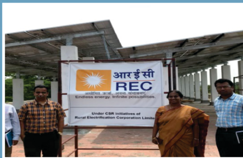
Installation of solar PV plant on campus of IIT Madras to reduce carbon footprint and promote green energy in the campus
